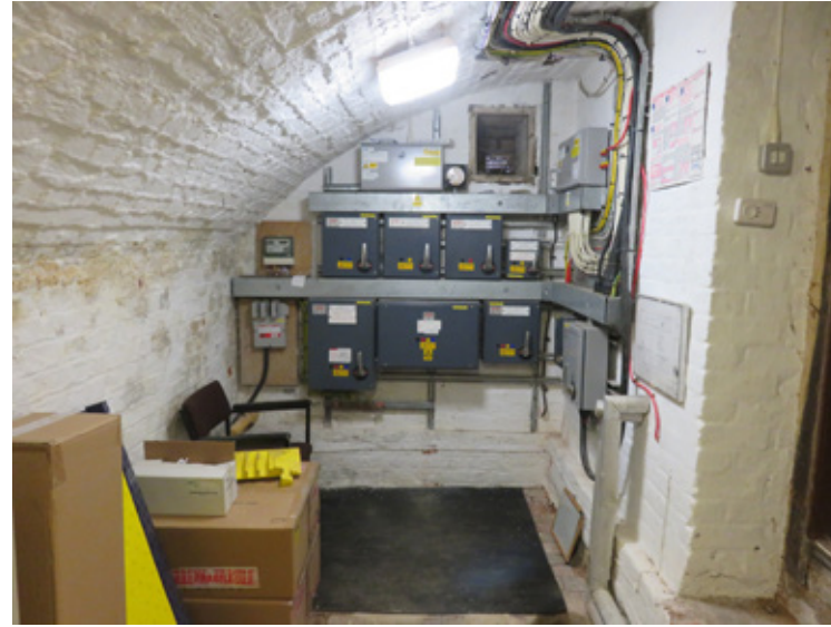
Figure 27 Interior of the brick vault on the lower-ground floor, beneath the portico, looking north.
