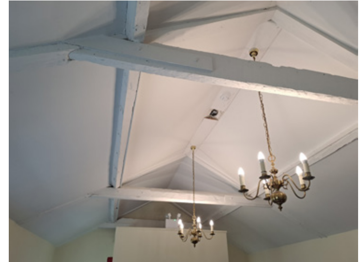
Figure 14 Rafters in the northern wing, upper-ground floor.
