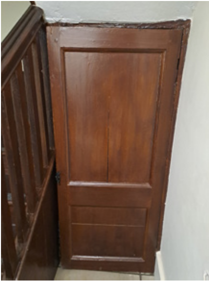
Figure 25 Door to under-stairs cupboard on the lower ground floor.
