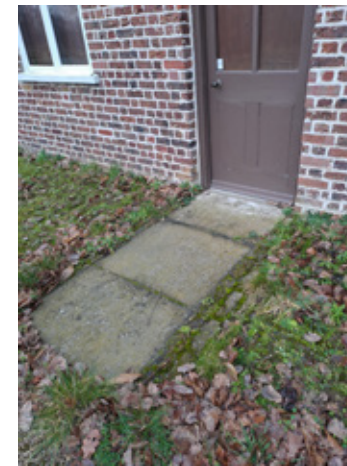
Figure 08 Paving laid to improve access to The Temple in the late 1990s
