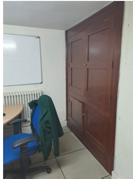
Figure 29 Modern joinery spanning a previous opening into the single-storey extension to the north, removed in the 1950s.
