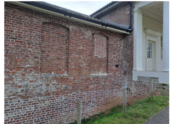
Figure 69 The west elevation of the north wing in 2023. The earth built up around the portico originally extended further backwards to meet the brickwork.
