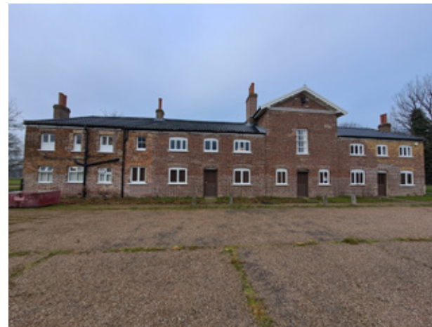
Figure 07 The east elevation of The Temple. On the left are the nineteenth century extensions
