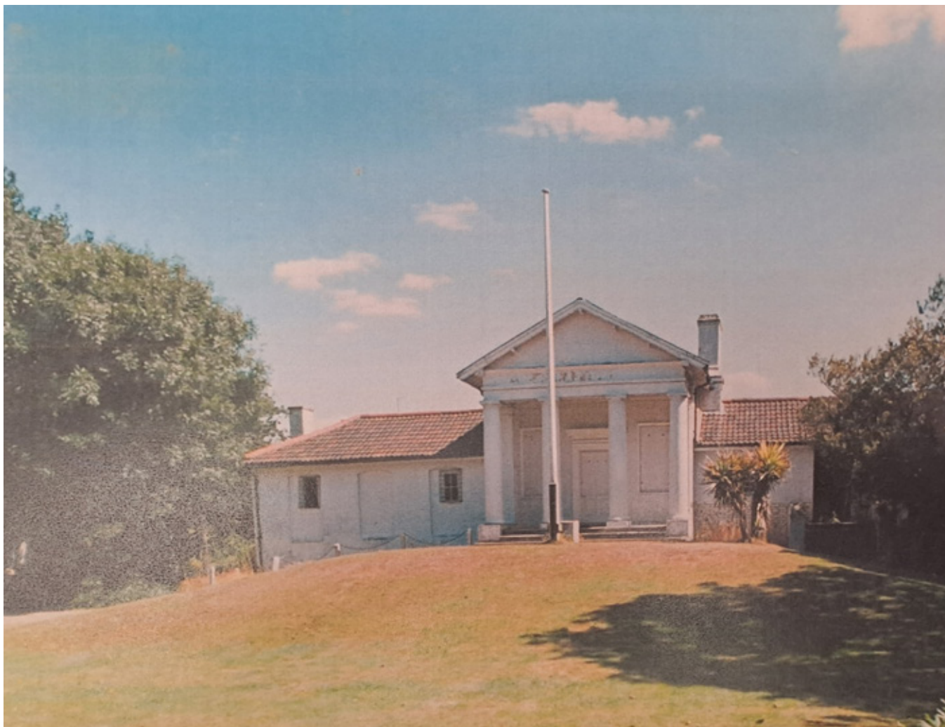
Figure 59 A photograph of the west façade of The Temple in the early 1990s. The late nineteenth century openings in the blind windows can be seen on the left, as can the twentieth century flight of steps and door leading to the first floor on the right of the portico. City of London Corporation, HB/TEM/16.
