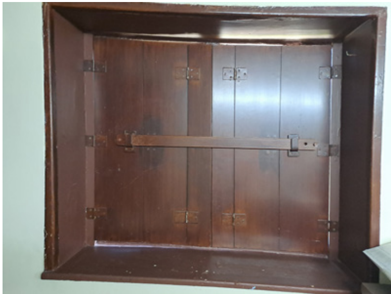
Figure 28 Modern security shutters on the lower-ground floor.
