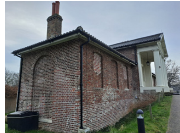
Figure 05 The Temple from the north-west. On the north elevation is the large blind archway dating from the 1990s. The areas of infill within the blind windows on the front elevation date from the early 1990s, when later nineteenth-century windows were removed. Note the earth sloping away from the front elevation up towards the path; originally the earthen mound continued to meet the brickwork.
